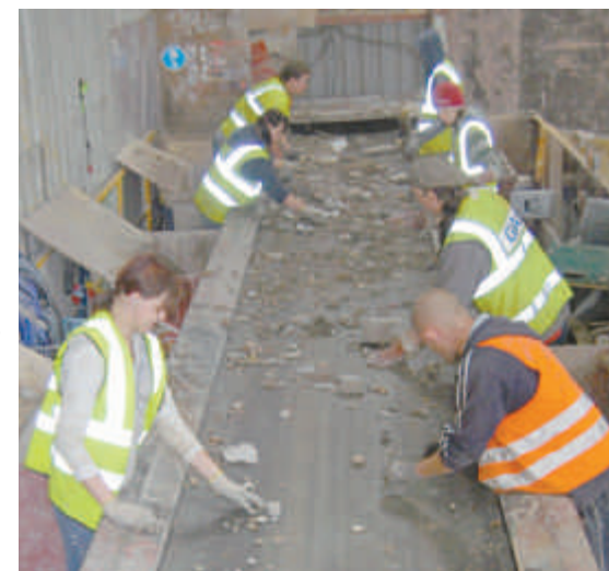
At work on the MRF - the materials recycling facility at the TBS site at Waterston
